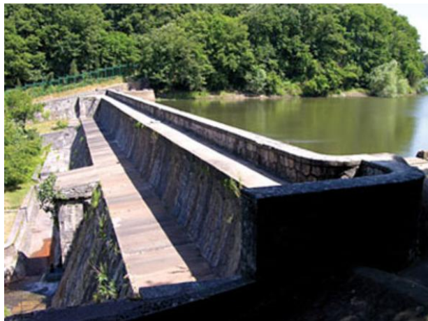
Figure 2 Topuz Bend Dam
